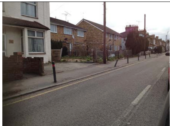
6. Cowley Mill Road, looking east, bollards that have been hit
